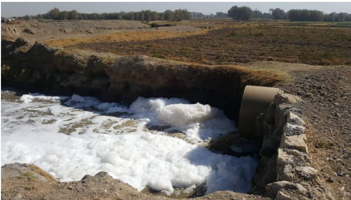
Fig. 3: The open earth canal of the treated wastewater.
